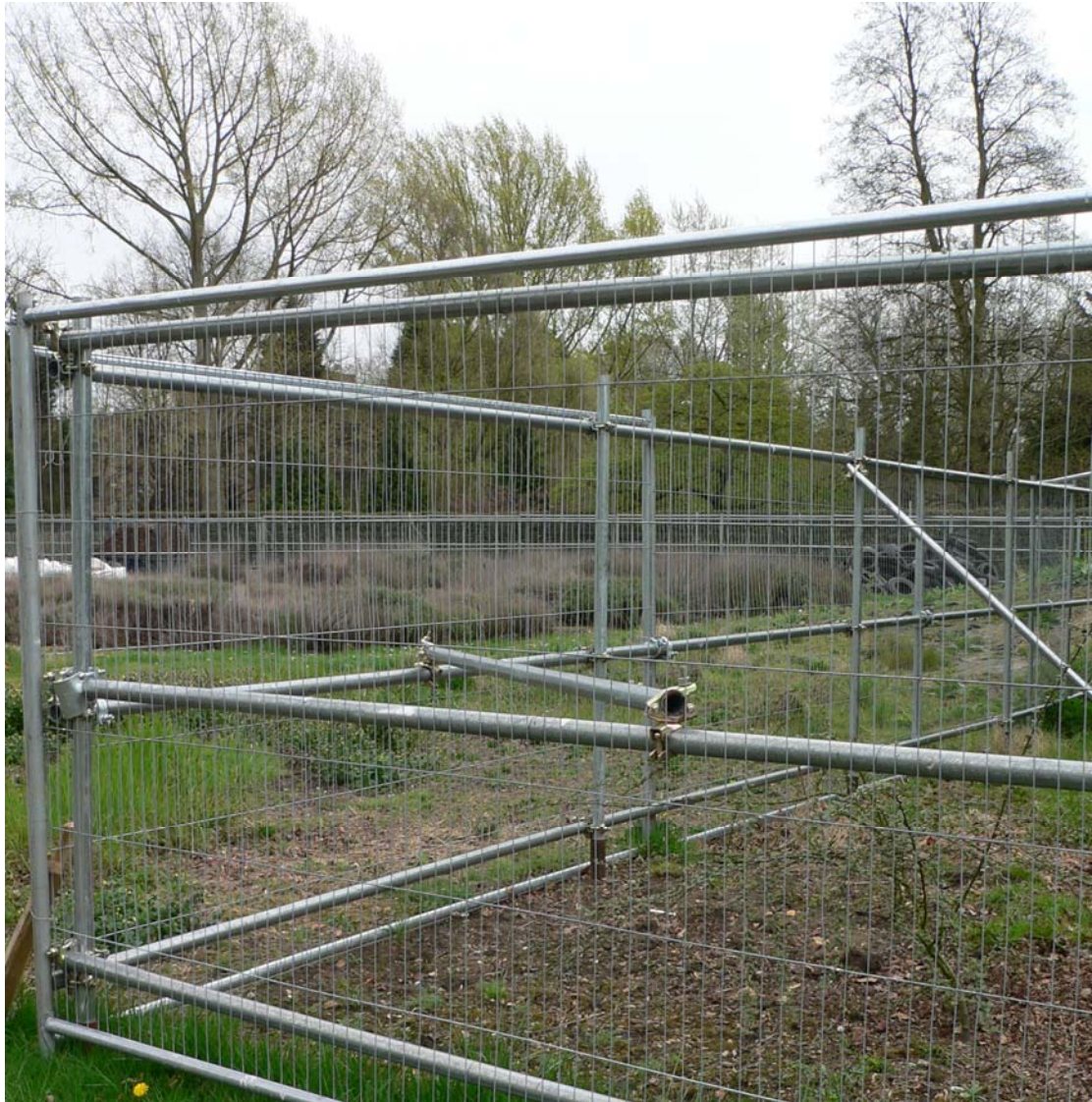
Detail of corner cross-bracing: part of protection for Liquidambar orientalis
